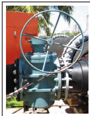
Cam-Centric® Plug Valve with worm gear actuator
