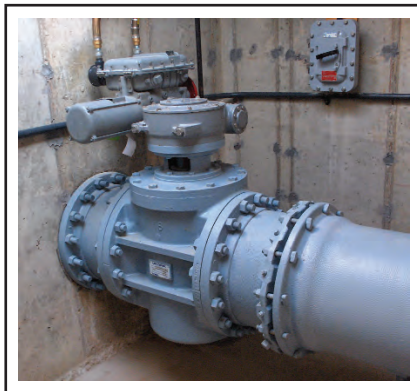
Cam-Centric® Plug Valve with motor actuator
